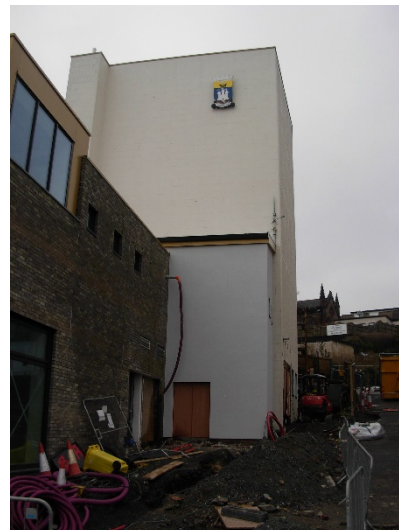
Northern elevation – fly-tower repointed and painted, new build sections (bottom left) and groundworks in preparation for new loading bay
