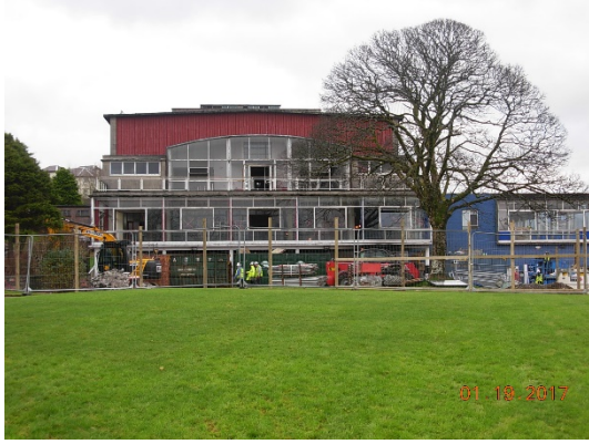
The southern elevation from Castle Gardens
