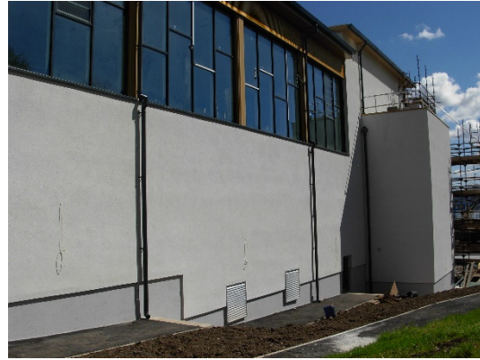
Western elevation – new double glazing, cladding and insulated render
